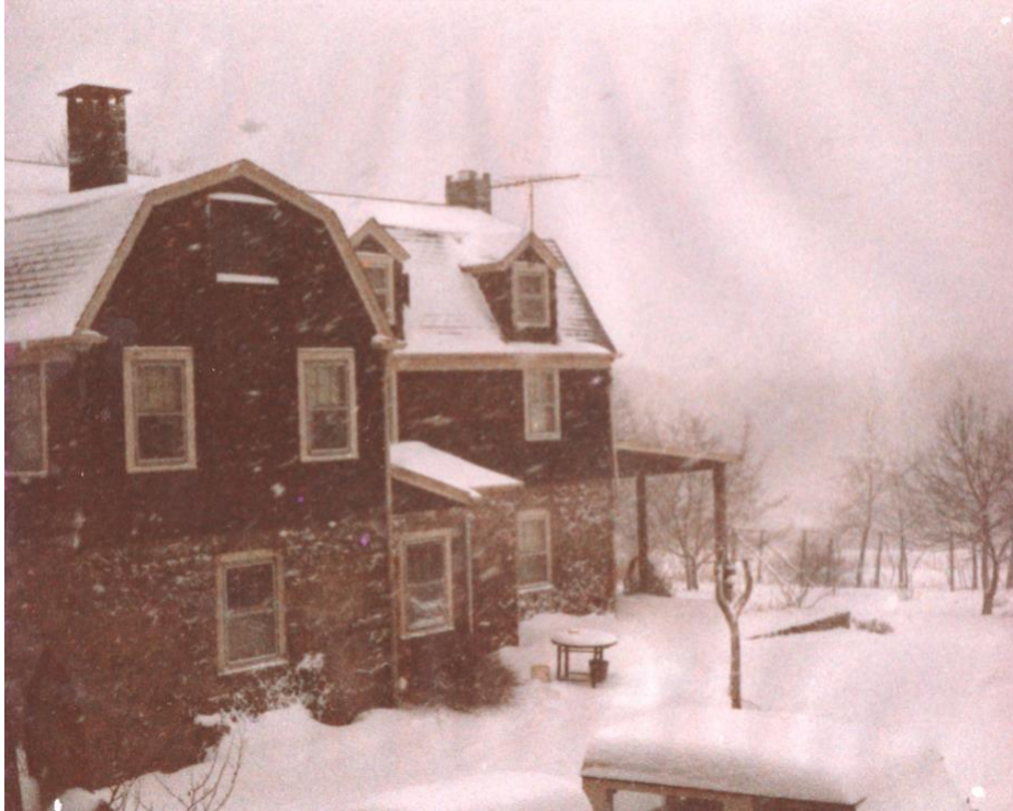
Rear (north) side of the house showing gambrel roof. Porch faces west. Historical photo; date unknown.
