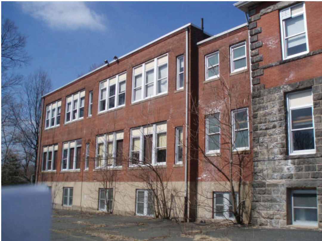
East façade of the southern most addition
