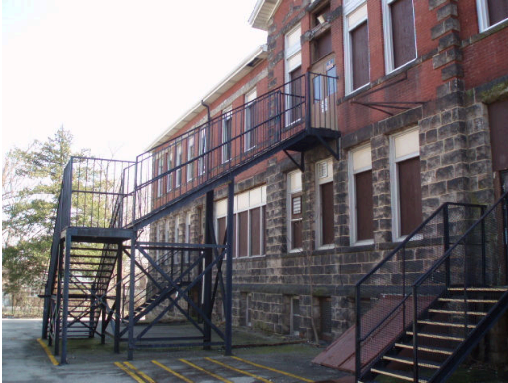
View of the rear (west) façade
