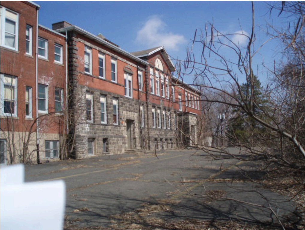
Front façade view from the southeast
