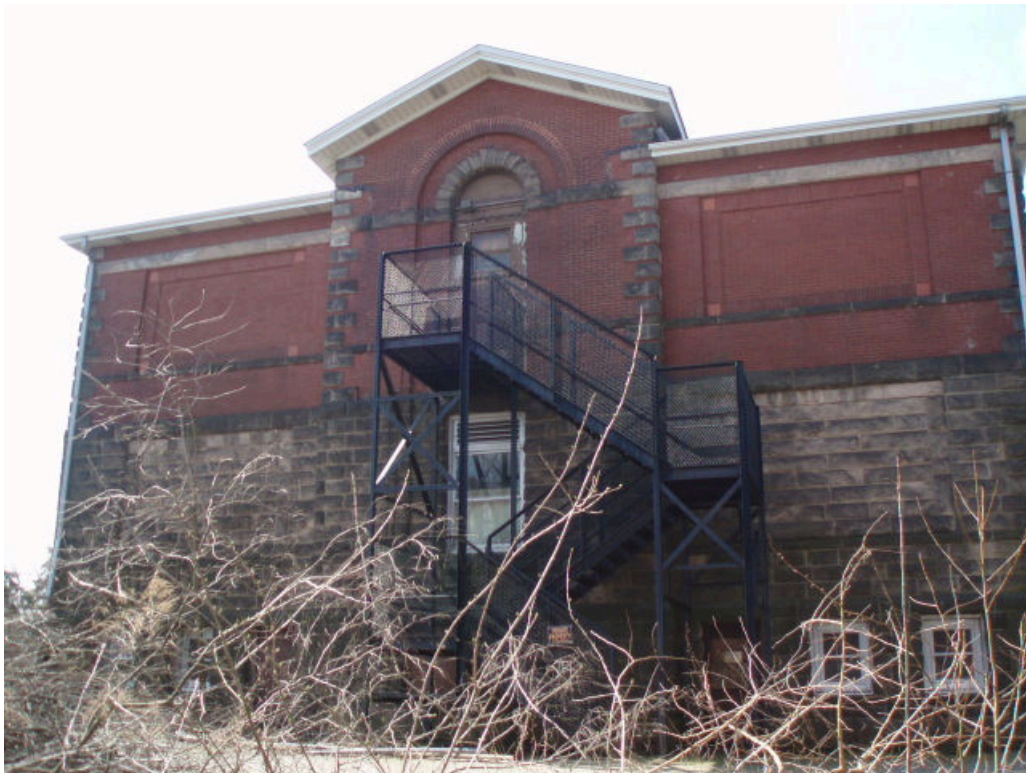
View of the north façade
