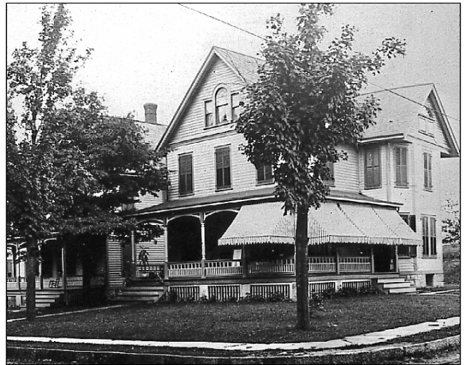
An early-20 th -century photograph documents the correct placement of awnings on a house to provide shade to a porch.
