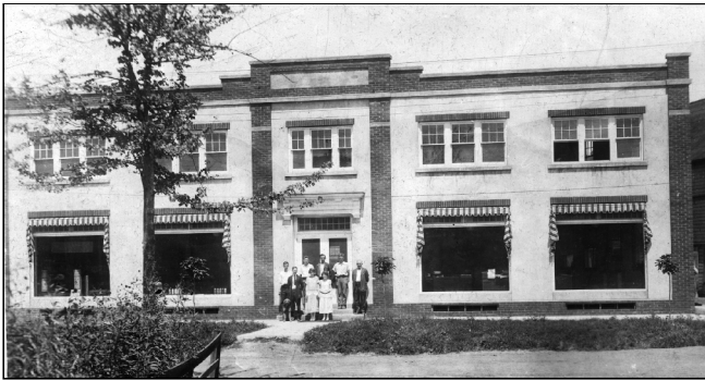
An early- 20 th -century photograph shows that the Demarest Hardware store had traditional striped awnings over display windows.
