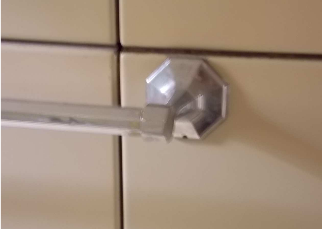
Fig. 92 – Original towel bar, photo taken looking north, June 2017.
