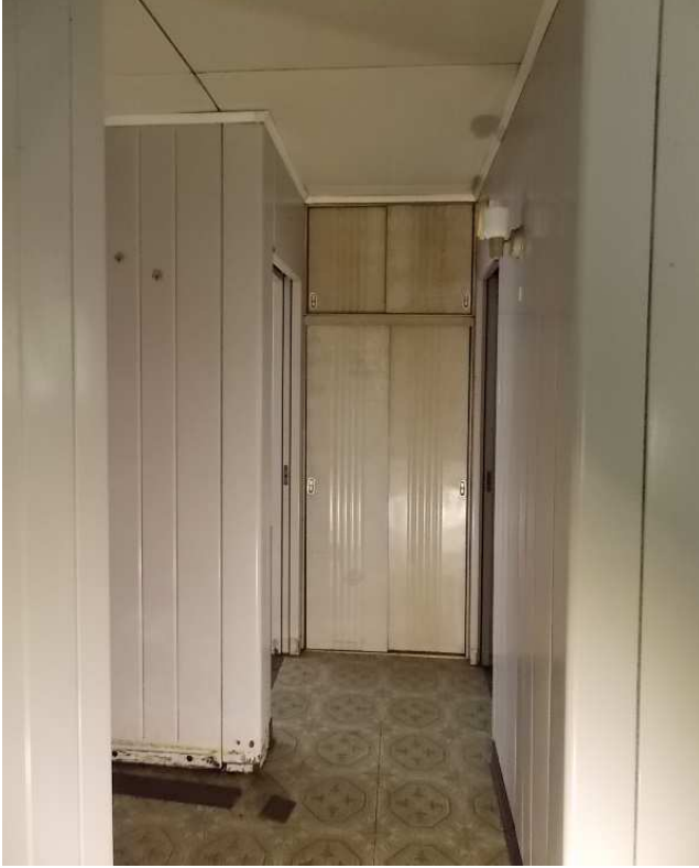
Fig. 82 – View of Hallway looking north with linen closet doors closed, photo taken June 2017.
