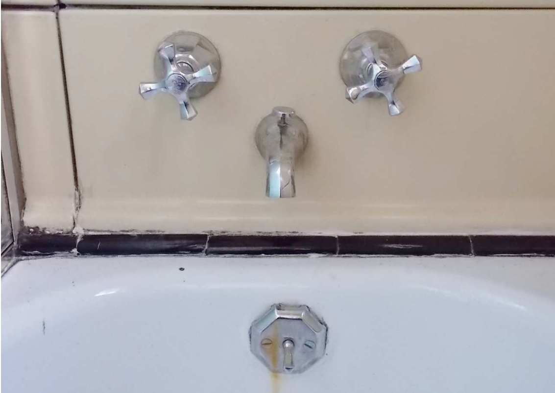
Fig. 90 – Original faucets, knobs, and cleanout. The black ceramic tile was added later, probably to conceal rust damage. Photo taken looking south, June 2017.
