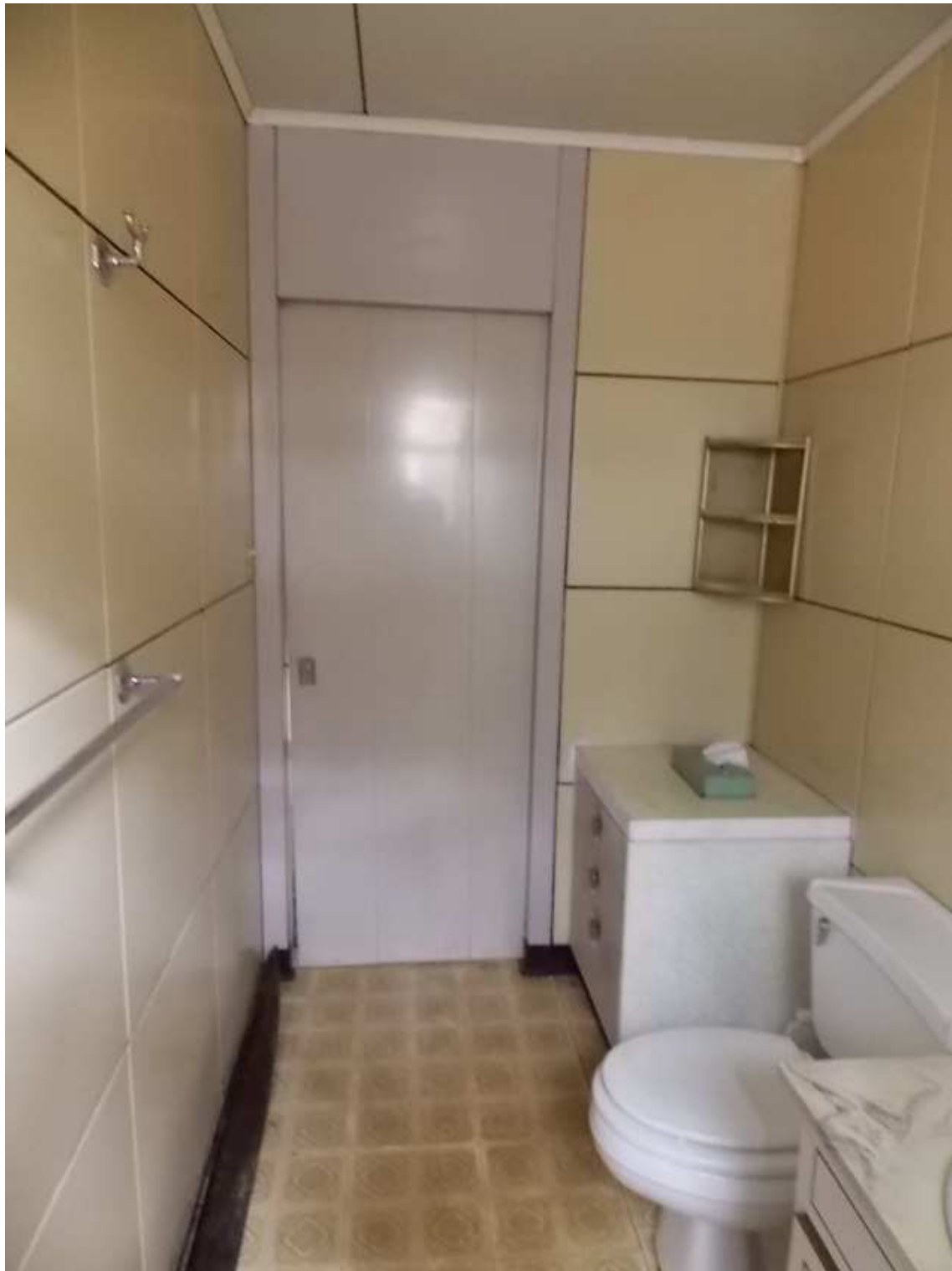
Fig. 87 – View of Bathroom looking east toward Hallway, photo taken June 2017. Note the original pocket door.
