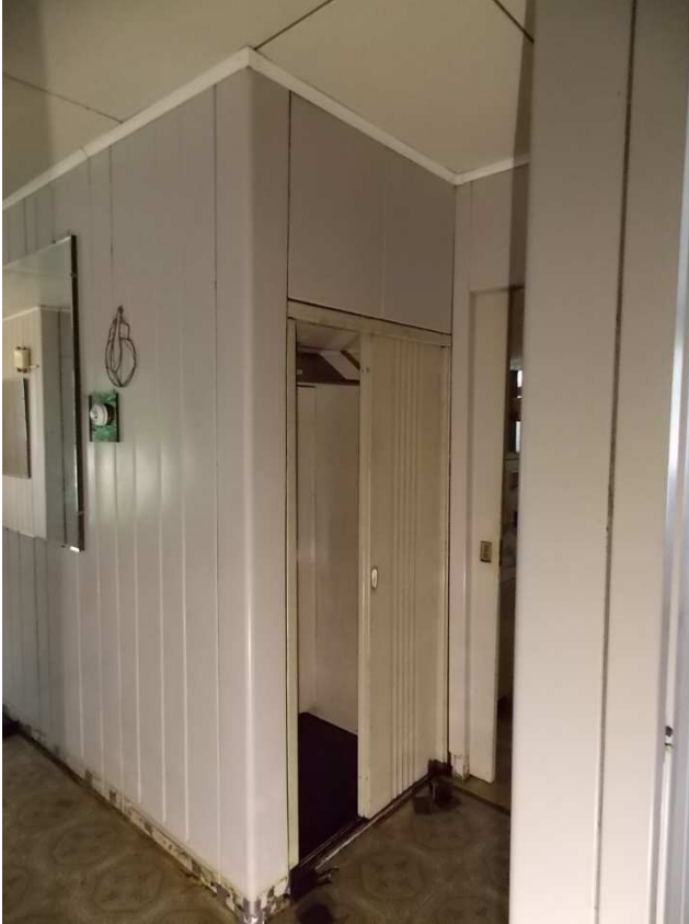
Fig. 80 – View of Hallway looking south toward guest closet, photo taken June 2017.
