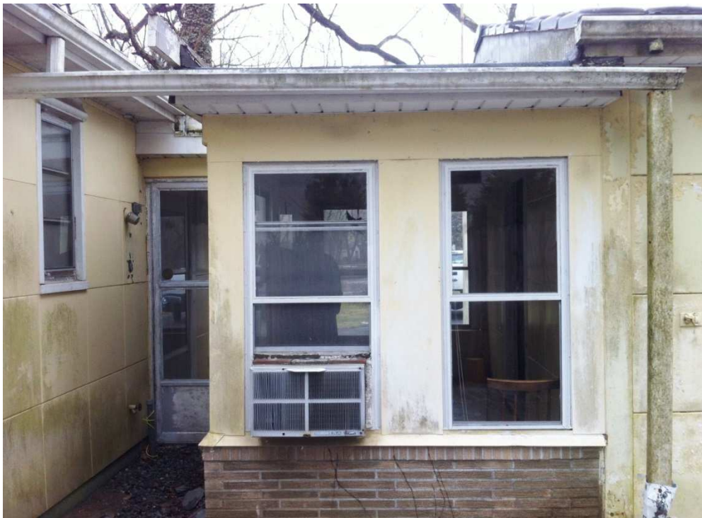
Fig. 52 – View of breezeway rear, photo taken looking south, March 2017.
