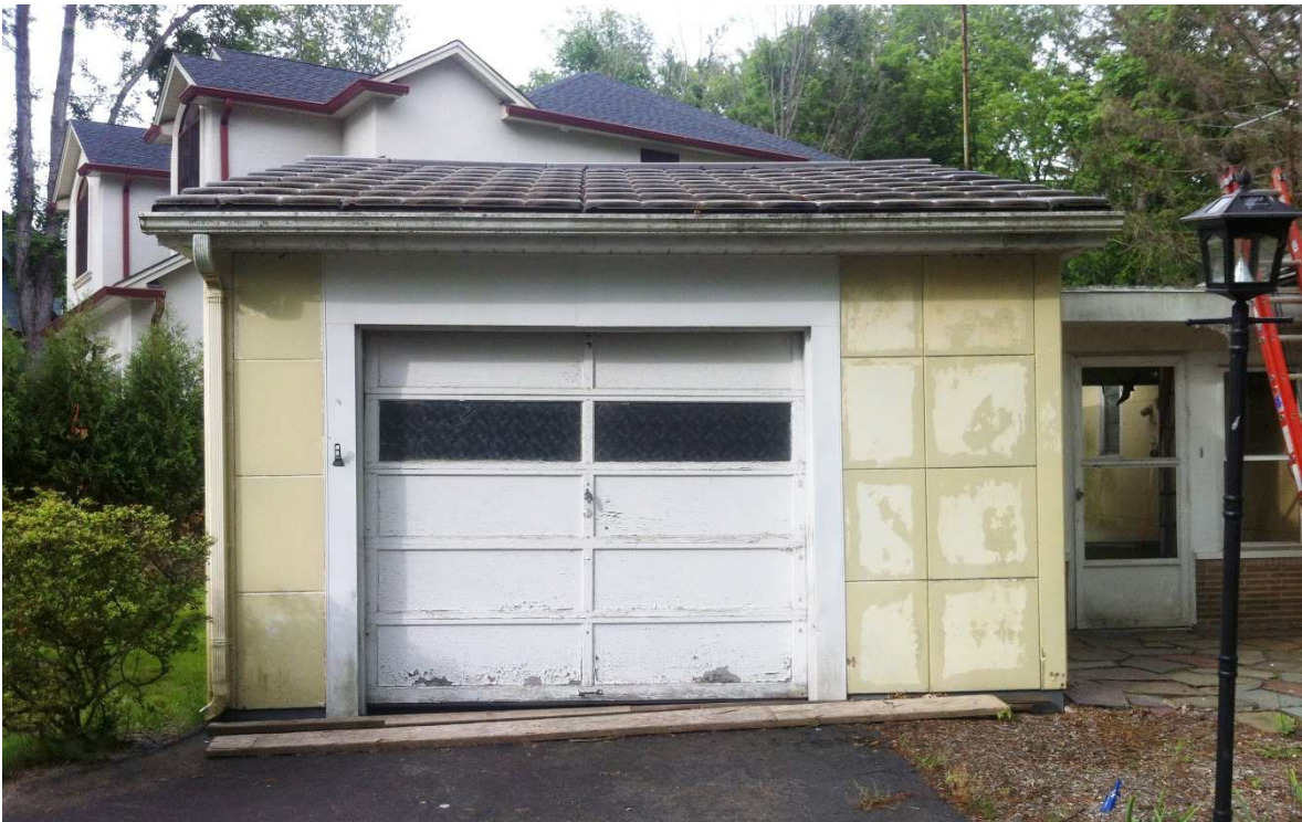
Fig. 17 – View of front of garage looking north, photo taken June 2017.
