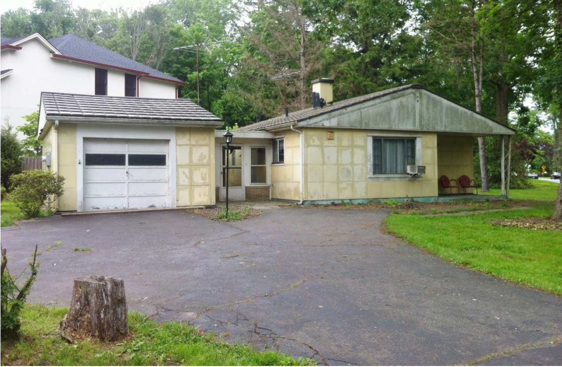
Fig. 10 – The asphalt driveway requires repair and sealing. The stump adjacent to the driveway should be removed and a new tree planted in its place. Photo taken looking east, June 2017.
