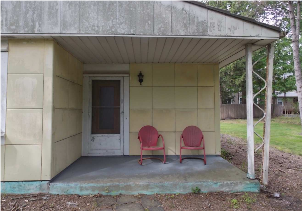
Fig. 7 – The flagstone walkway to the front porch should be re-graded to create a handicapped accessible path from the driveway to the front door. The remaining foundation area should be left exposed, photo taken June 2017 looking east.
