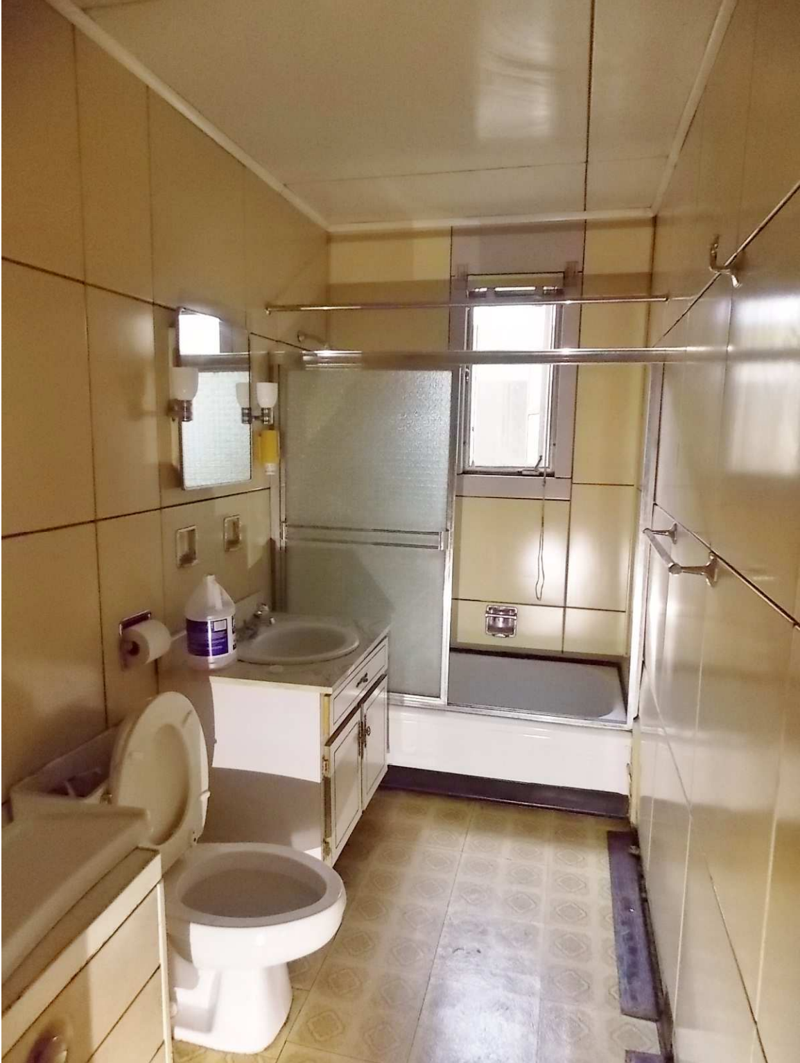
Fig. 86 – View of Bathroom looking west from Hallway, photo taken June 2017. Note the glass shower doors which have been added.
