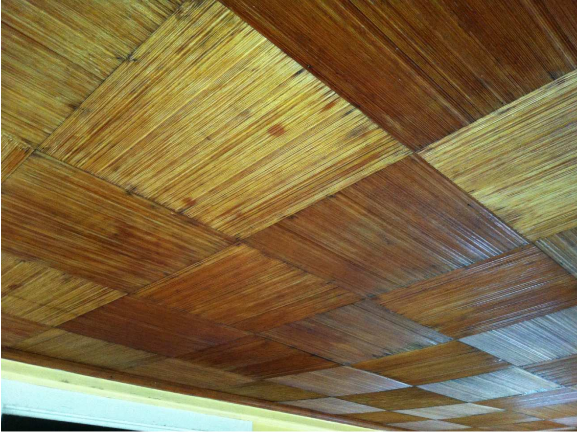
Fig. 55 – View of breezeway ceiling, photo taken looking east, June 2017.
