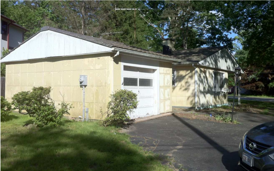
Fig. 115 – View of Garage looking east, photo taken June 2017. Note new electrical service location.
