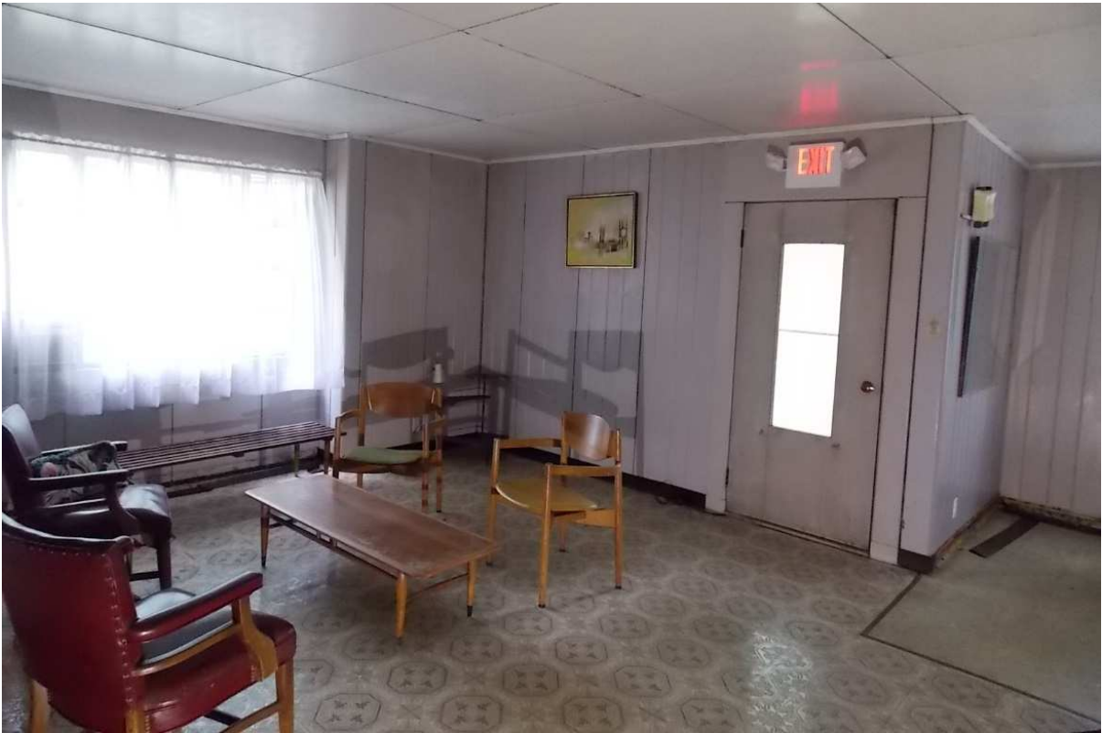
Fig. 77 – View of Living Room looking south from the Hallway, photo taken June 2017. Note the new Exit / Emergency lighting.
