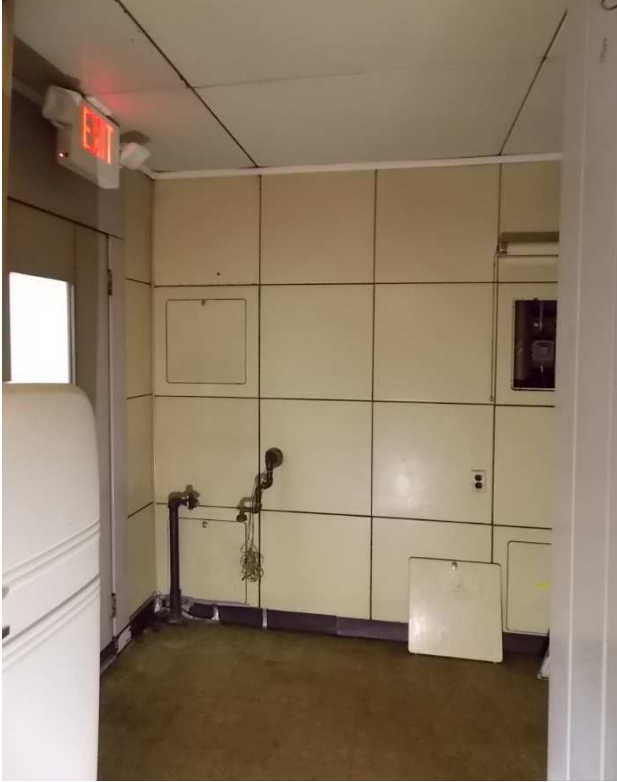
Fig. 63 – View of utility wall from Kitchen looking north, photo taken June 2017.
