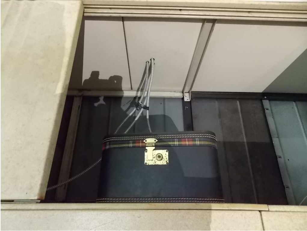
Fig. 99 – Recent electrical wiring was routed through the closet ceiling, photo taken looking south, June 2017.
