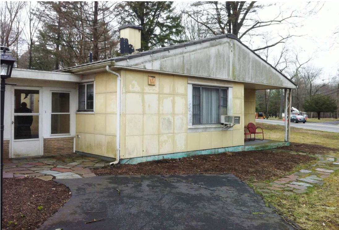
Fig. 11 – The flagstone paving in front of the breezeway should be re-laid, photo taken looking southeast March 2017.
