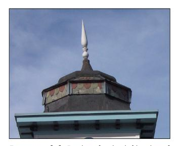
**Recommended:** Retain and maintain historic rooflines, character-defining roof materials, and historic roof features as exemplified by this picturesque polygonal-shaped tower roof with colored shaped slates and terminating finial.
