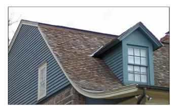
**Recommended:** Use a roof material that is compatible with the historic architecture. The wood shingles on this early stone house reflect the traditional roofing material of the late 18<sup>th</sup> century.
