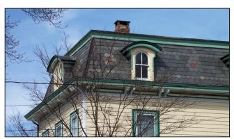
**Recommended:** Retain and maintain characterdefining historic rooflines such as this mansard roof, roof materials such as these multi-colored patterned slates, and original historic roof features such as the bracketed overhanging eaves and elliptically arched dormers.
